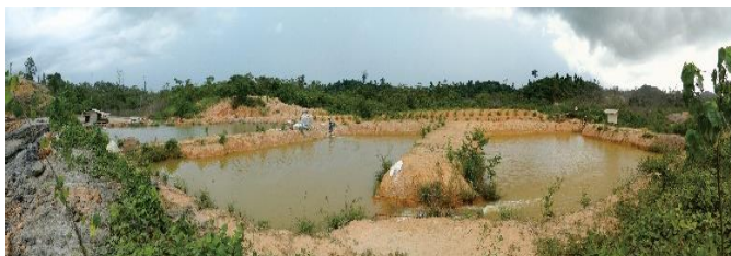
Figure 3: Example of AMD handling process in a sedimentation pond with neutralizing material, followed by flow through an open channel into a swamp as a surface water reserve.
