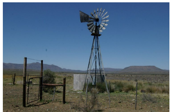
Plate 1: Typical example of a windmill that pumps the underground water into the associated reservoir for storage commonly found in the Karoo.
